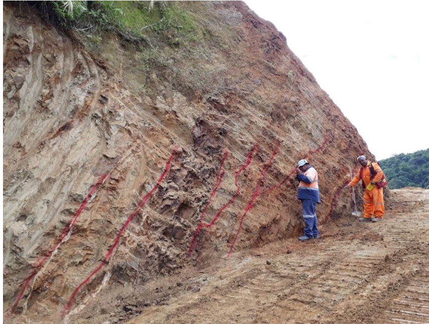
Figure 1: Current benching from Banana Creek prospect, SPL 1512, exposing intensely altered mineralised structures with sulphides rich veins and visible specks of bornite with magnesium oxide. Note that 5g/t Au was sampled from this area prior to benching.
