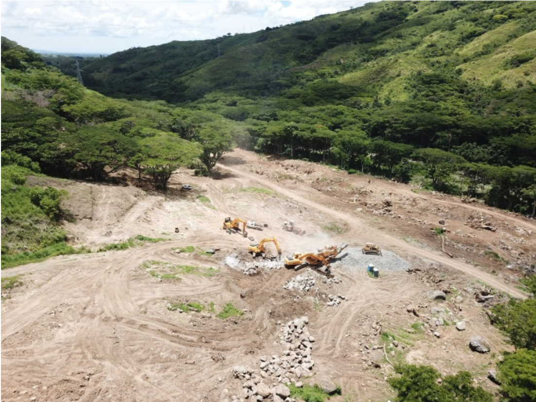
Aerial View of Tuvatu Plant Site: Bulk Earthworks Construction Underway
